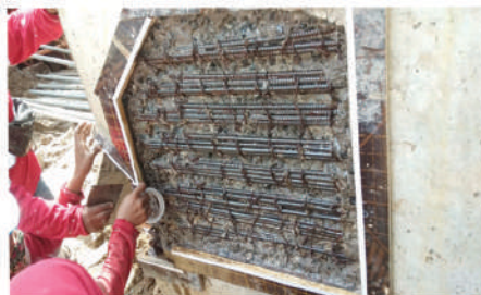
PIER GIRDER & PILE CAP REPAIR - CRACK & SPALLING CONCRETE REPAIR Asian Grain Corporation - City of Naga, Cebu
