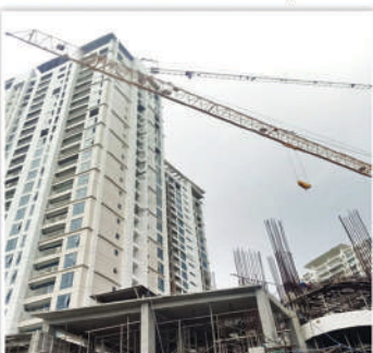
MIDPOINT TOWERS, MANDAUE CITY
