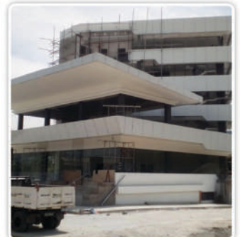
COMMERCIAL BLDG., BANAWA, CEBU CITY
