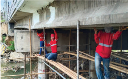
BRIDGE GIRDER STRENGTHENING - INSTALLATION OF CARBON FIBER PLATE Pakigne Bridge, Pakigne, Minglanilla, Cebu
