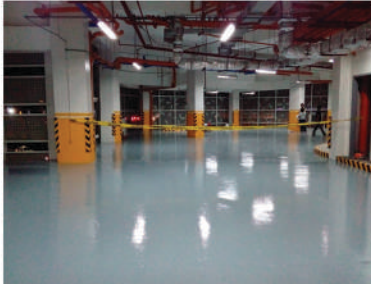
ONE MADISSON PLACE TOWER 1 & 2 (PARKING DECK) SELF-LEVELLING EPOXY COATING Ilo-Ilo City
