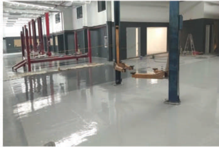
NISSAN GATEWAY MOTORS (SERVICE AREA) SELF-LEVELLING EPOXY FLOOR COATING V. Rama Ave., Cebu City
