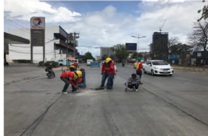
EPOXY CRACK INJECTION - NORTH ROAD, MANDAUE RECLAMATION AREA Mandaue City, Cebu
