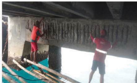
PIER GIRDER & PILE CAP REPAIR - CRACK & SPALLING CONCRETE REPAIR Asian Grain Corporation - City of Naga, Cebu
