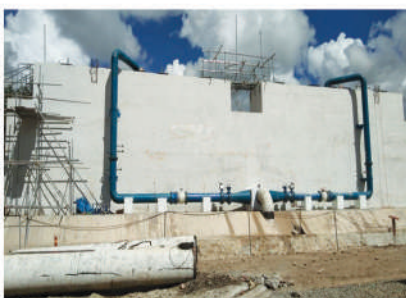
CRACK REPAIR - PULSATOR CLARIFIER TANK Manila Waters Project, Carmen, Cebu
