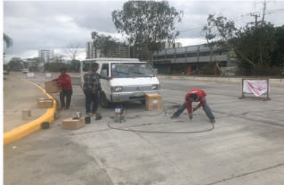
EPOXY CRACK INJECTION - NORTH ROAD, MANDAUE RECLAMATION AREA Mandaue City, Cebu
