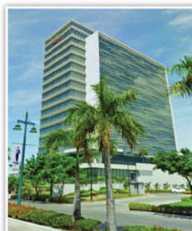
COURTYARD MARRIOTT HOTEL, ILOILO CITY
