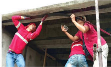
BRIDGE GIRDER STRENGTHENING - INSTALLATION OF CARBON FIBER PLATE Pakigne Bridge, Pakigne, Minglanilla, Cebu
