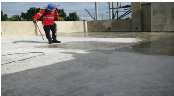
BORRAMEO COMMERCIAL BUILDING - Roof Deck Pinamungahan, Cebu 400.00 sq.m.
