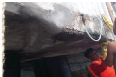
CRACK REPAIR & CONCRETE SPALLING REPAIR - BERTHING/MOORING STRUCTURE Asian Grain Corporation, City of Naga, Cebu
