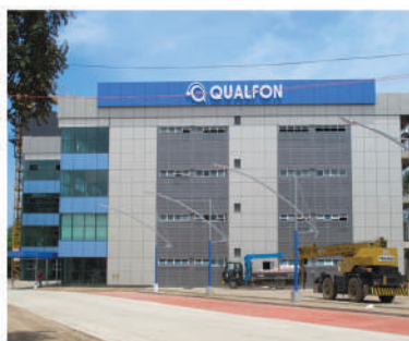
LinkSY BLDG. QUALCOM SITE 2 Dumaguety City
