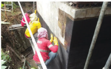
SHEAR WALL - Carbon Fiber Strengthening School Building , Cebu City
