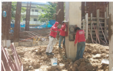
COLUMNS & RETAINING WALLS - HONEYCOMBS REPAIR The BLOQ 2 Building, Sikatuna Street, Cebu City
